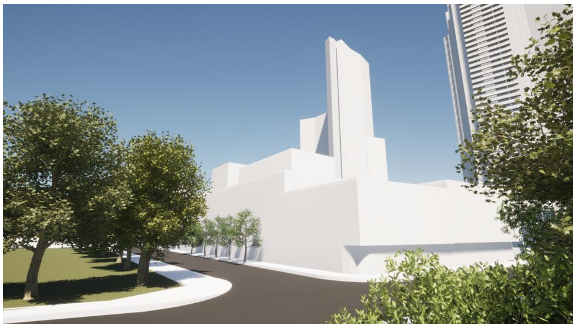
Figure 5 – Concept design render looking southeast from corner of Marsden Street and Market Street, Parramatta (noting this is at a maximum height of 28m and excludes any Design Excellence bonus)
